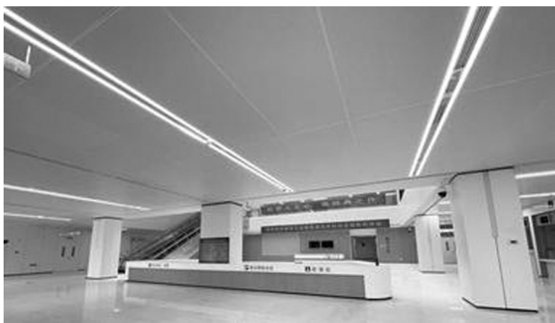
顶面施工工艺龙骨安装
